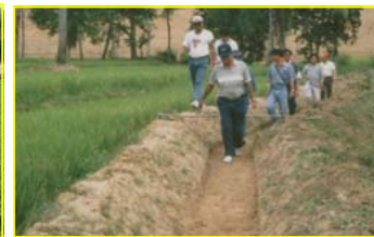
Earth canal structure
