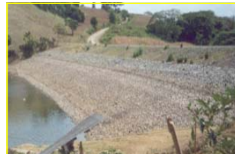
Embankment (modified homogeneous earthfill)
