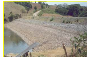
Embankment (modified homogeneous earthfill)
