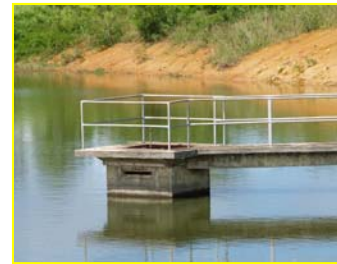
Intake control structure
