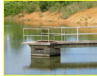
Intake control structure
