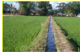
Lined canal structure
