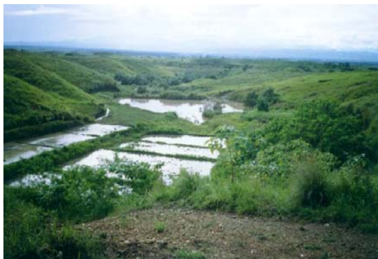
The Small Farm Reservoir (SFR) is an earth dam structure use to trap and store rainfall and runoff (Photo: BSWM)
